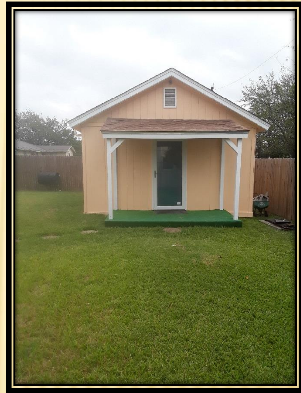
View of the existing Accessory Structure
