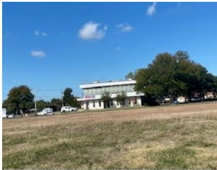
West of the subject property
