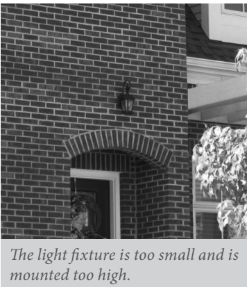
The fixture obscures architectural detail and is mounted too high.
