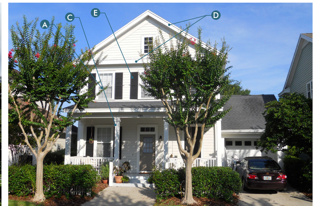
A Regular, repetitious composition of windows; B Side gable roof; C Ornamentation at entry stoop or porch; D Shallow eaves and rake with a simplified classical cornice; E Louvered or raised panel shutters; F Gabled Dormer
