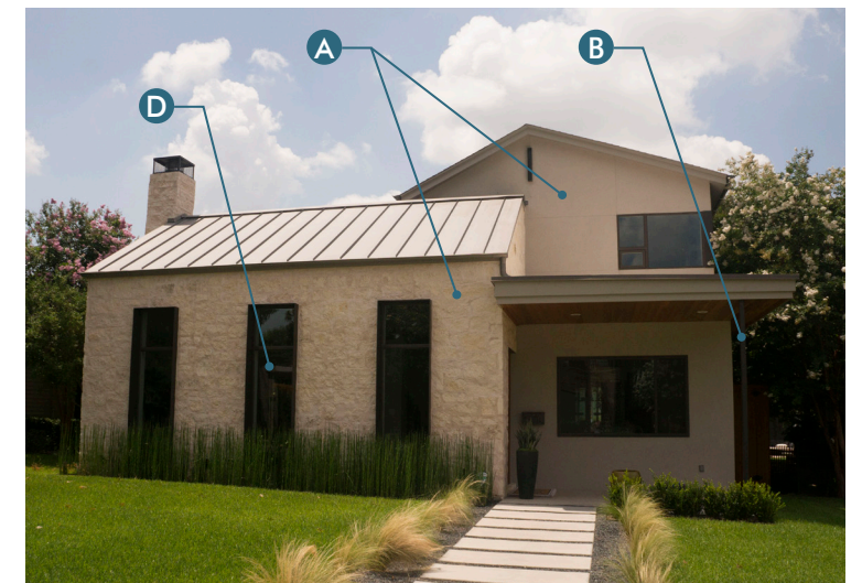
A Combination of multiple cladding materials or material applications; B Simple exposed structural members; C Shallow pitched shed roof; D Single pane fixed window; E Modern interpretation of traditional form
