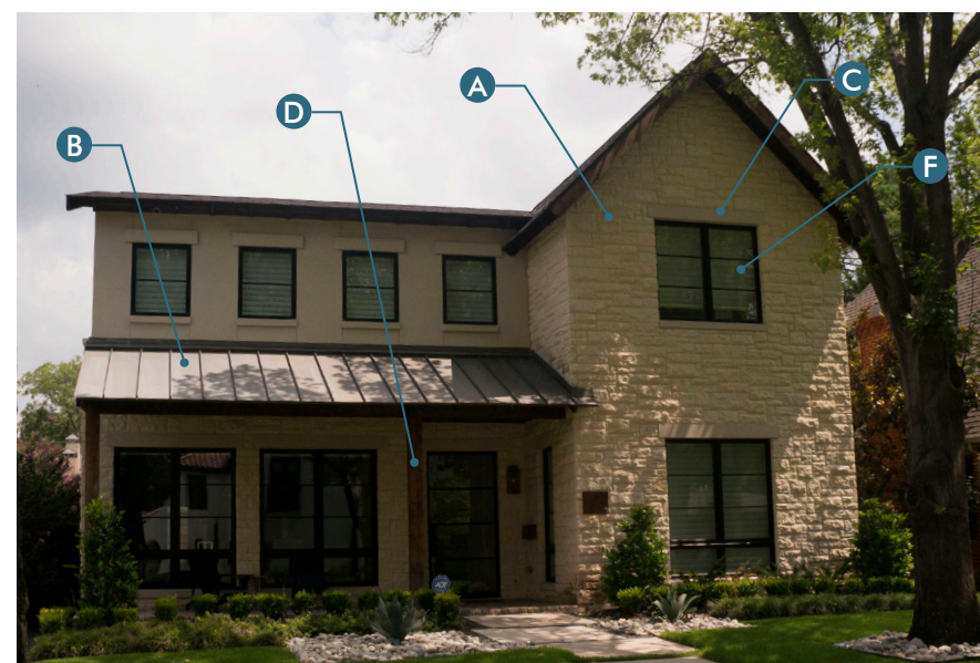
A Local stone cladding; B Standing seam metal roof; C Heavy timber or monolithic stone lintels; D Simple square porch posts; E Post brackets; F Modern horizontal window panes; G Traditional vertical window panes
