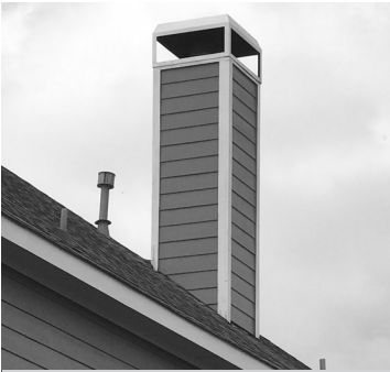
Siding should not be used as a finish material for a chimney.
