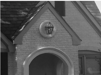
The fixture obscures architectural detail and is mounted too high.
