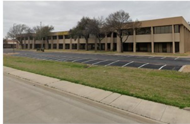
Looking west of the subject property |
