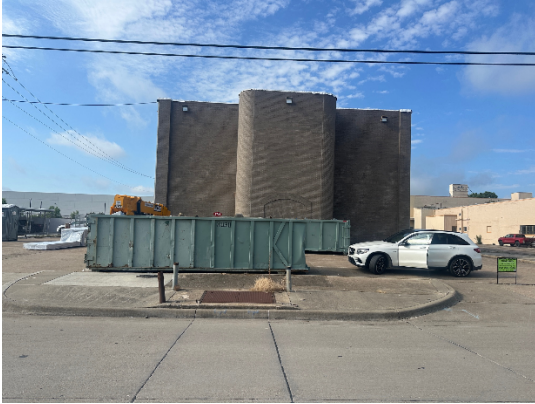
View of subject property facing south.
