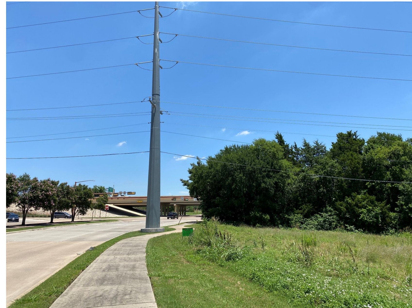
Looking North toward State Highway 190.
