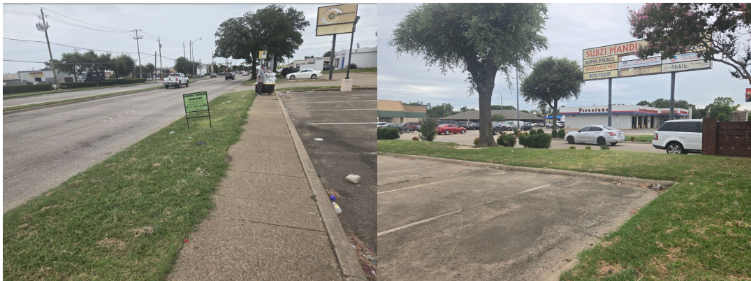
View of Buckingham Road facing east
