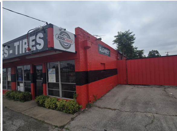
View of site facing southeast up close to the signage
