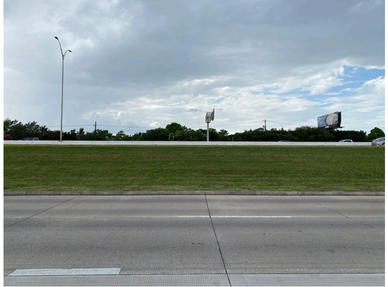
View from the subject site looking at Interstate 30.
